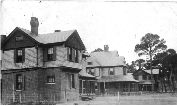
Hog Island Lighthouse Keepers' Dwellings c. 1897
