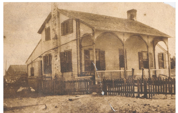
Smith Island Lighthouse Keeper's Residence
